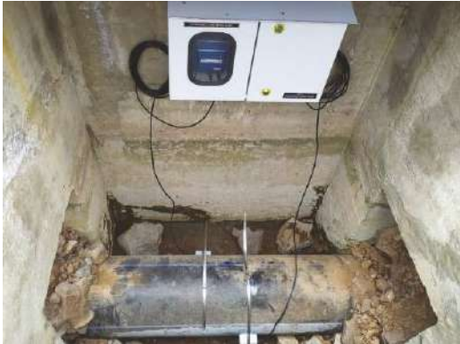
Installation of Clamp-On Type Ultrasonic Flow Meter
